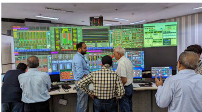
Observing Real-Time Control Room Monitors
